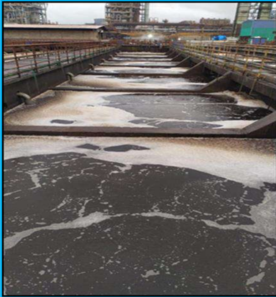
Pictorial view of Aerobic and anoxic treatment of BOD Plant Coke oven -2
