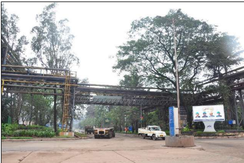
Green belt near LD Plant and internal road
